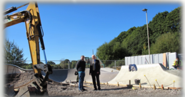
Cllr Chris Thom and Cllr Alan Dowden overseeing the progress of the new skate park at Knightwood Leisure Centre
